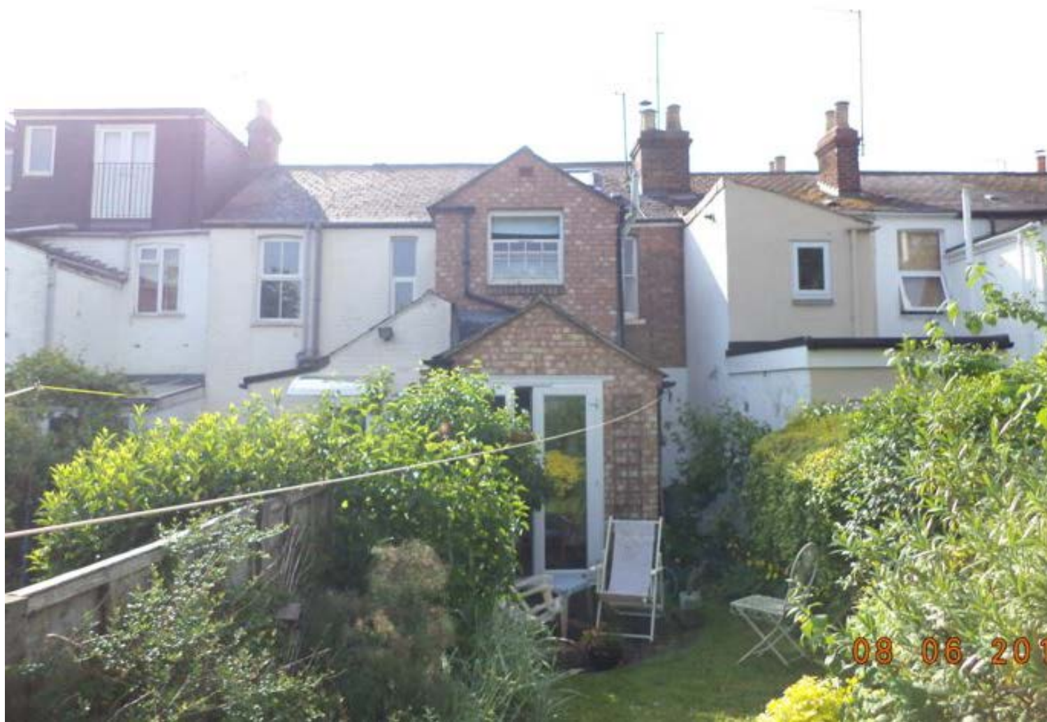
Rear Elevation 9 Union Street
